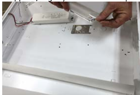
Installing LED Strips in Fixture With TEK Screws
